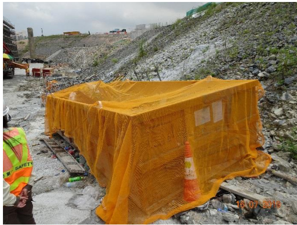
Exposed surface was covered by cement mortar
