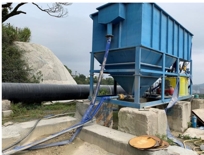
Q5: Wastewater treatment facility 11 cu. m. + AquaSed of 60 cu. m. per hour
