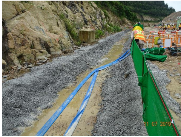
Perimeter channel to collect site surface
