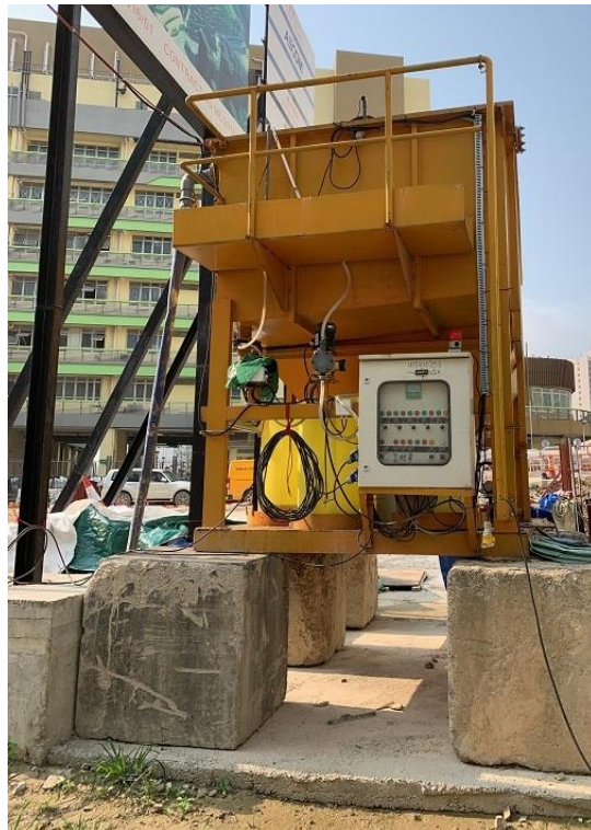
Q7: Wastewater treatment facility AquaSed of 60 cu. m. per hour
